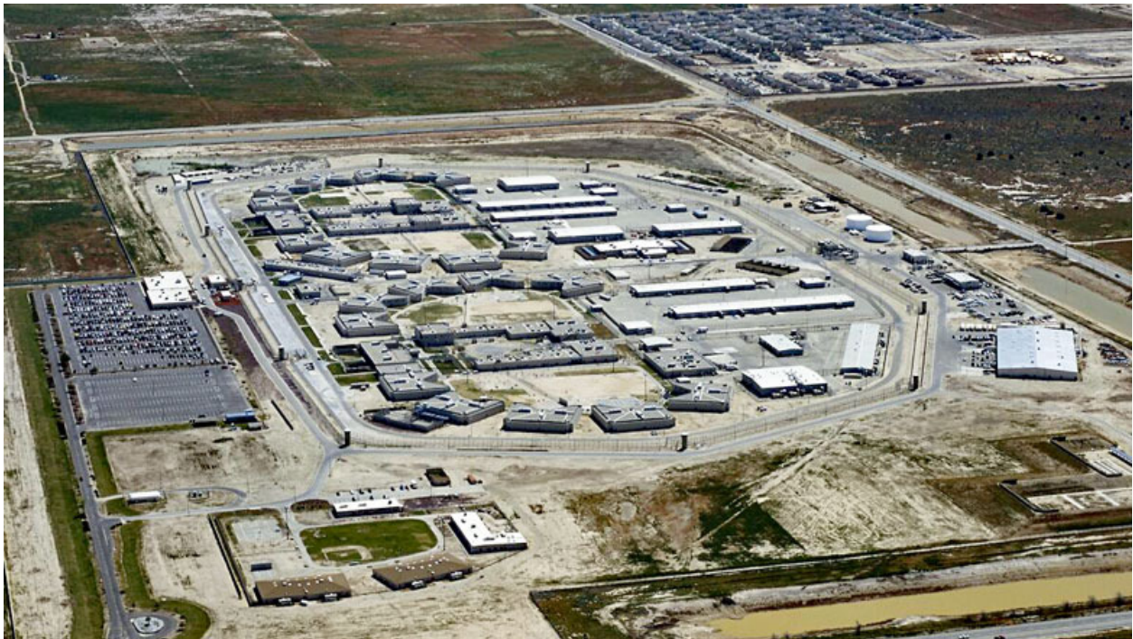
California State Prison, Los Angeles County in Lancaster, CA
