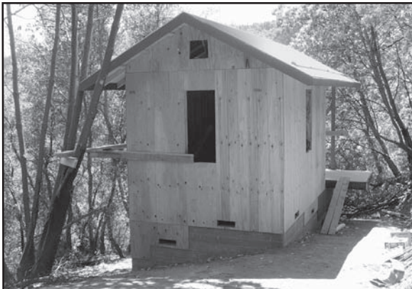
New monk's cabin under construction
